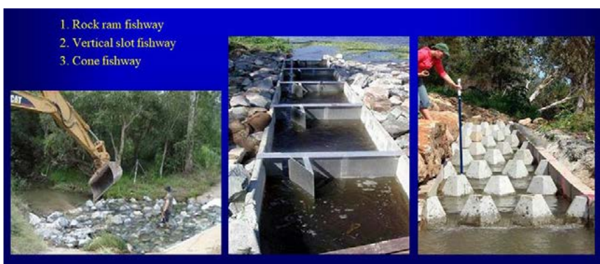
Figure 12. The form of fishway to use is another design challenge: whether a rock ramp fishway (left), a vertical slot fishway (centre) or a cone fishway (right).
