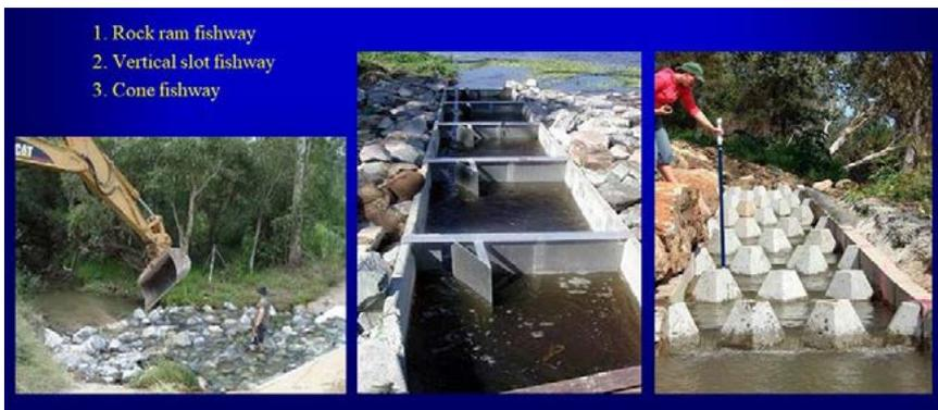
Figure 12. The form of fishway to use is another design challenge: whether a rock ramp fishway (left), a vertical slot fishway (centre) or a cone fishway (right).
