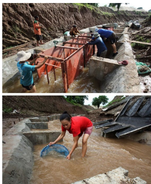
Figure 3. Fishway under construction at Xayaburi Dam on the Mekong River.
